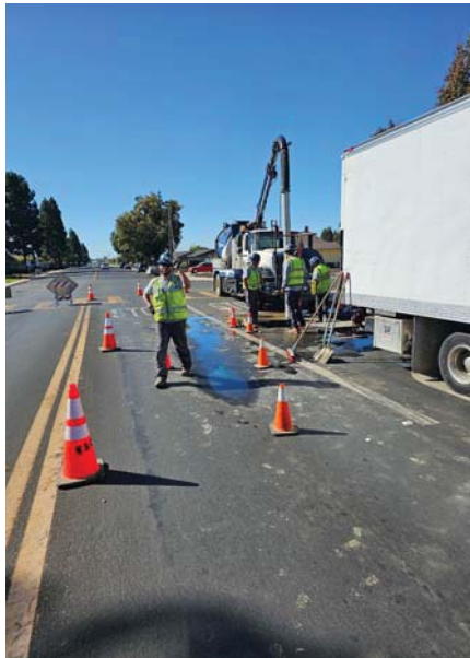
VacCon in use during line repair.
