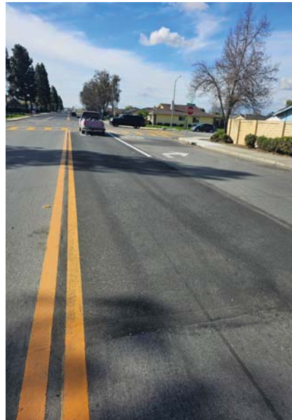
Completed asphalt repair.
